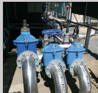
Gippsland Water Factory, Australia
