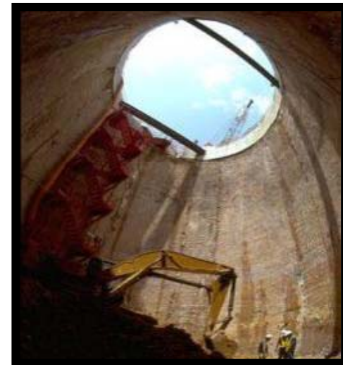
Deep Tunnel Sewerage System, Singapore
