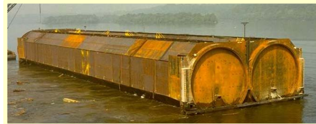
Fort McHenry Tunnel, Baltimore
