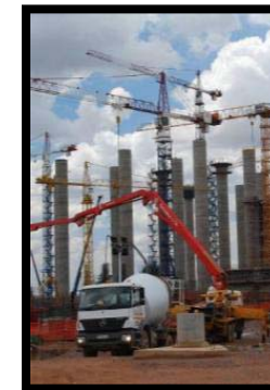
Medupi Power Plant, South Africa
