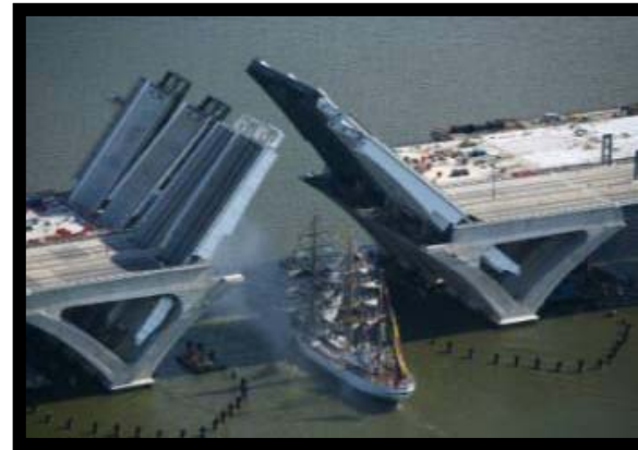
Woodrow Wilson Bridge, Maryland/Virginia
