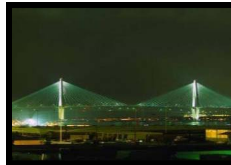
Arthur Ravenel Jr. Bridge, South Carolina
